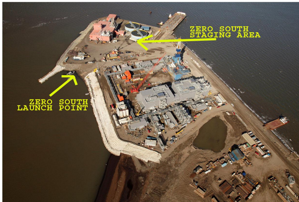
Oliktok Point in summer. The ZERO SOUTH PTVs were prepared for the sea ice near a water treatment plant which served as a wind barrier during final preparations. (Photo provided by State of Alaska, Department of Natural Resources)
