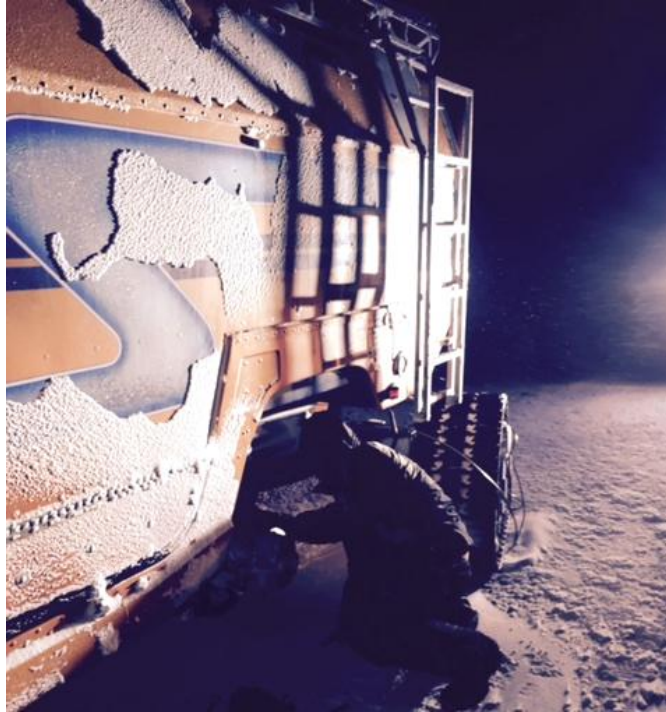
Braving -20° Fahrenheit and 20 MPH winds, Charlie Zacarias replaces a geared hub on PTV2. Component-level repair is necessary rather than attempting a rebuild in-the-field. (Photo by Nick Baggarly)
