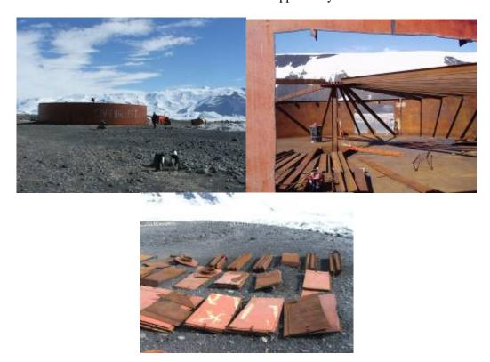
Figures 4,5 and 6. Fuel tank prior to dismantling; dismantling in progress; sections of fuel tank ready for helo lifting to the *Italica*.
